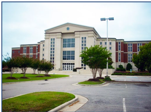
▲ Harnett County Courthouse.
