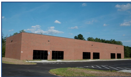
▲ Western Harnett Industrial Park
