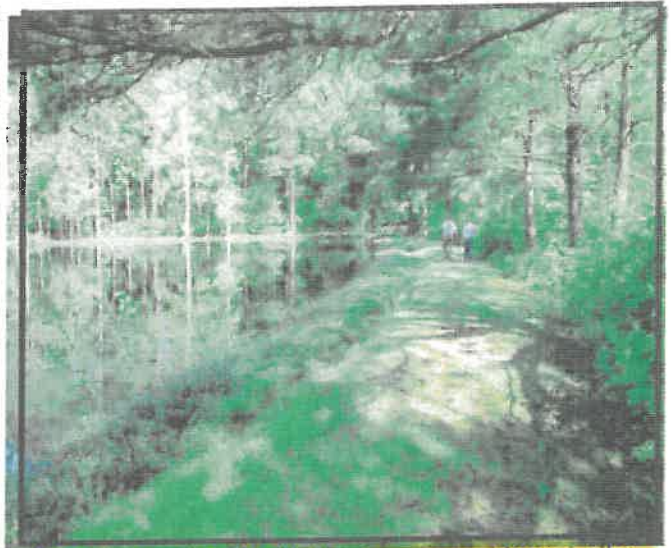
Pond dam & potential driveway looking at site
