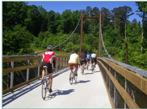
NW Harnett greenways are proposed to connect to the Wake County Greenway System
