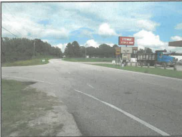
Elliot Bridge Road N. View
